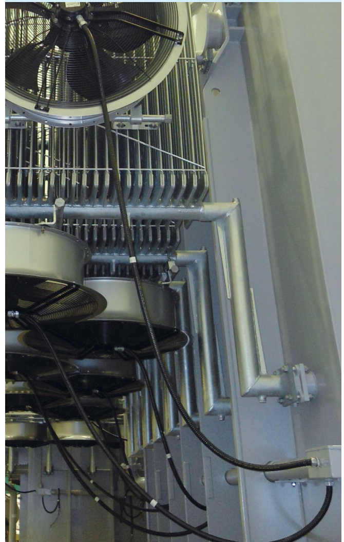
FIGURE 5. Top: The thermo–fluid dynamics simulation of the new design. Bottom: New collecting pipes design. In the new design, the pipes have been removed from their previous position circling exterior of the reactor. Instead, the pipes travel directly from the cooling fan and into the reactor itself.
