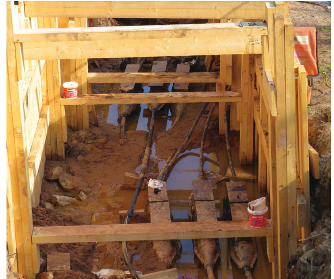
FIGURE 5. Photo of field joints being used to connect separate sections of cables together.
